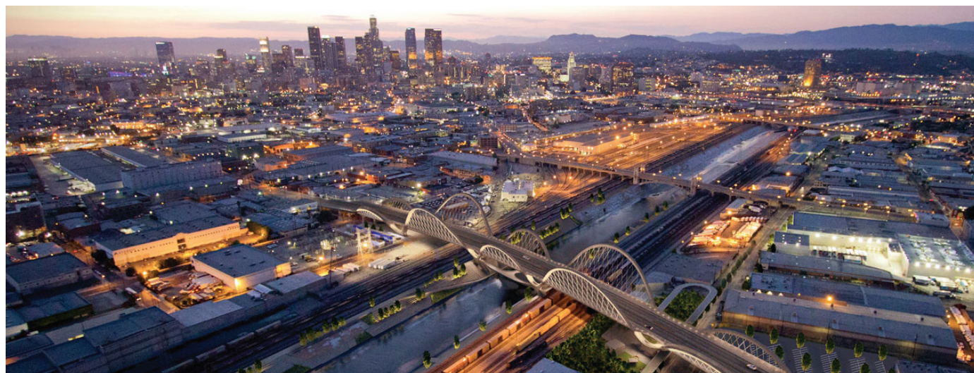
6th Street Viaduct, Los Angeles, USA.
