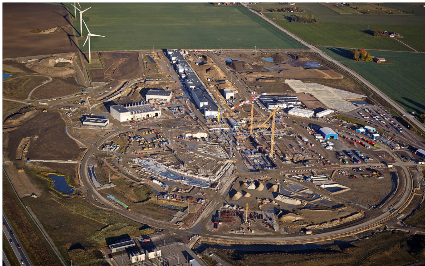
ESS Research Facility, Lund, Sverige.
